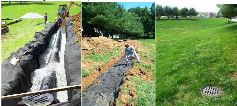
Figure 4: Example of Infiltration Trench Installation
